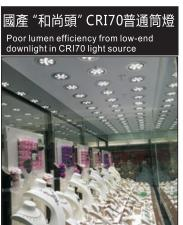
一般内地廠商的Led 燈具缺點:使 **用塑膠透鏡有多重疊影,影響視** 覺及腦神經 , 在歐洲已經不建議 使用,光輸值只有80流明/瓦以下 短期出現光衰,顯色只有70%以 下,影響展品的質感及留於平面化 General Chinese manufacturers provide multi-chips LED in 80lm/W and CRI70, resulting in overlapping shadow and affecting the visual feeling. They have not been suggested using in Europe.
